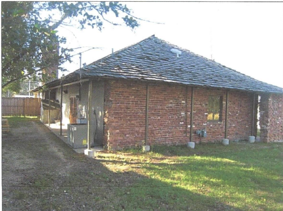
Rear view of office building
