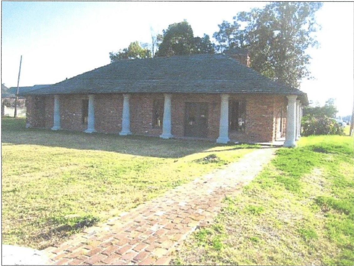
Front view of office building
