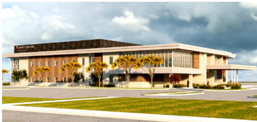
Now Under Construction
