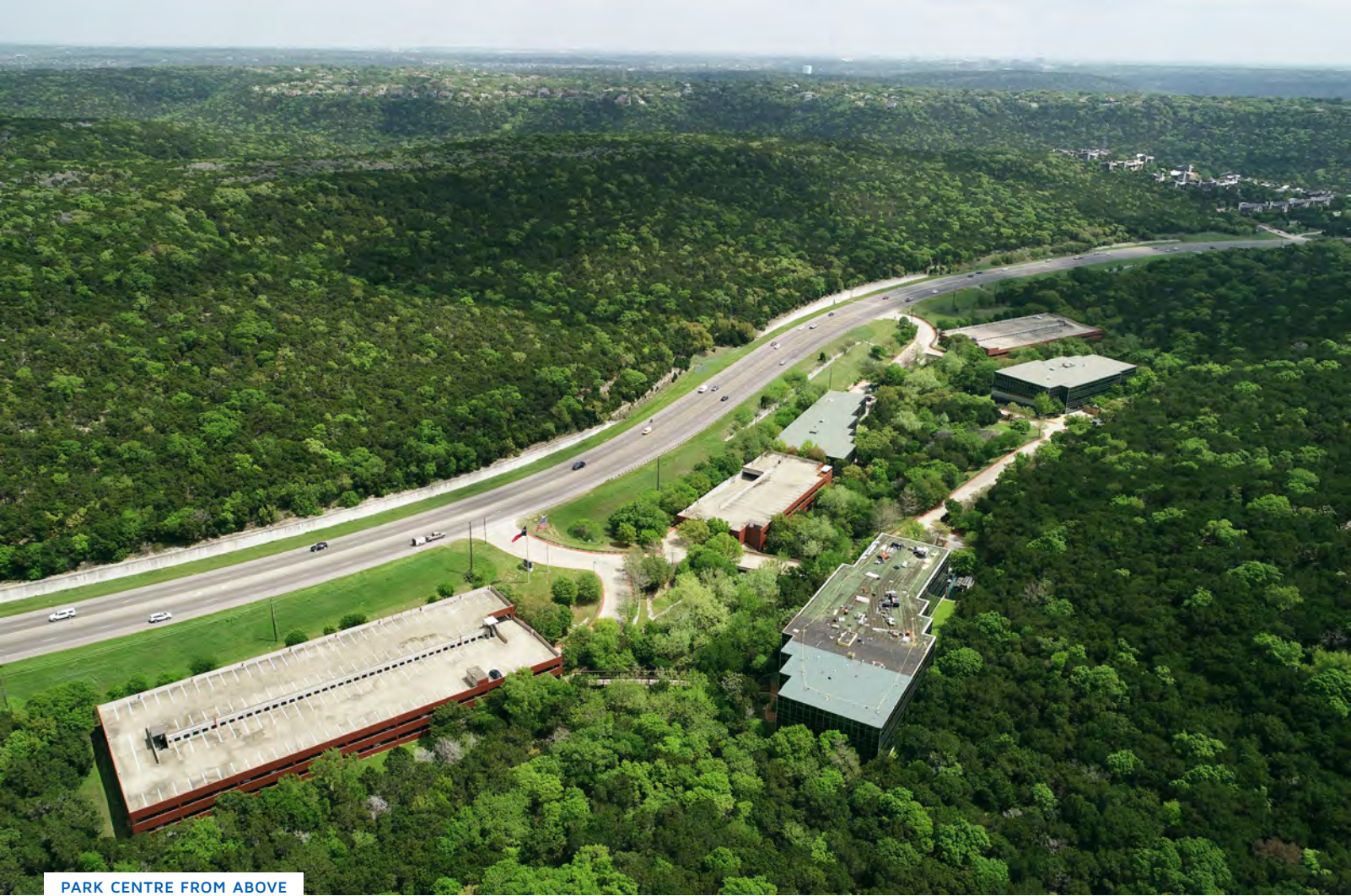
PARK CENTRE FROM ABOVE
