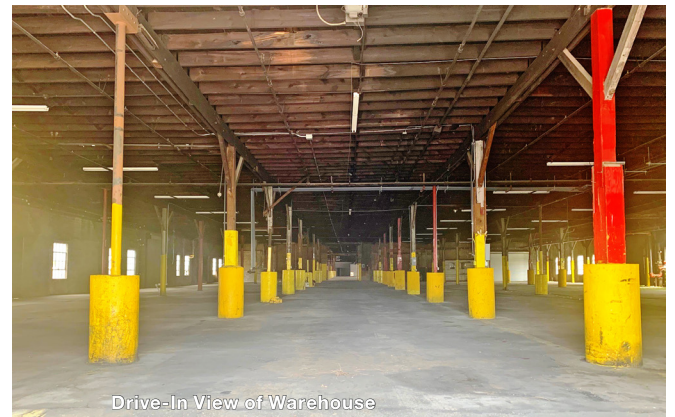
Drive-In View of Warehouse
