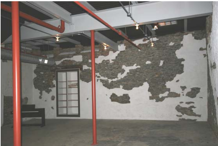
Interior Garden Level
