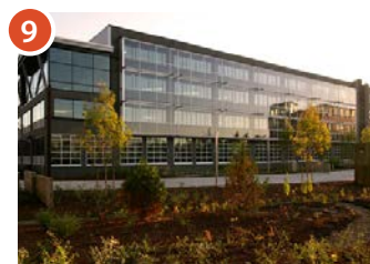
9 VIEWPOINT SOFTWARE HQ 1515 SE Water Ave. 90,000 SF Office Redevelopment
