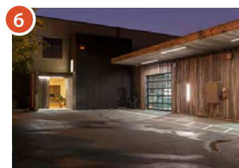
6 STUMPTOWN HQ 100 SE Salmon St. 37,000 SF Roasting, Training + Offices
