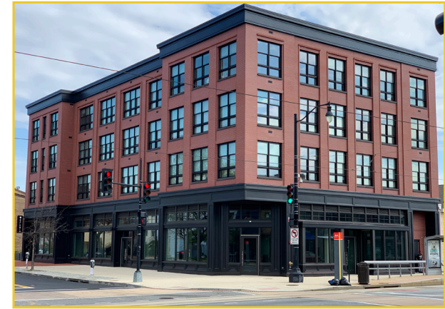
VIEW ALONG 13TH STREET NE
