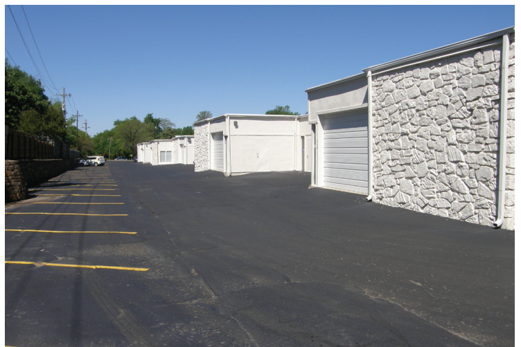
Back Section with New OH Doors
