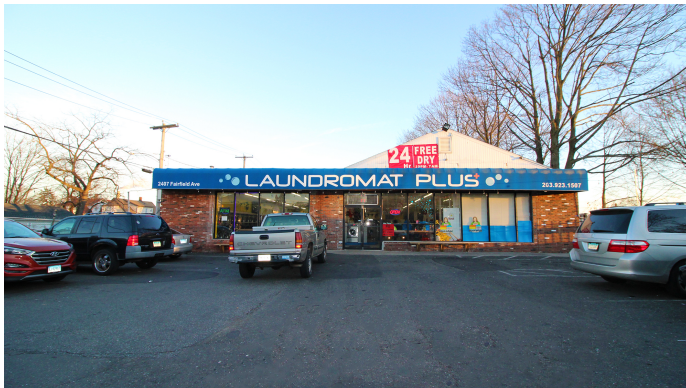
FULLY LEASED BUILDING
