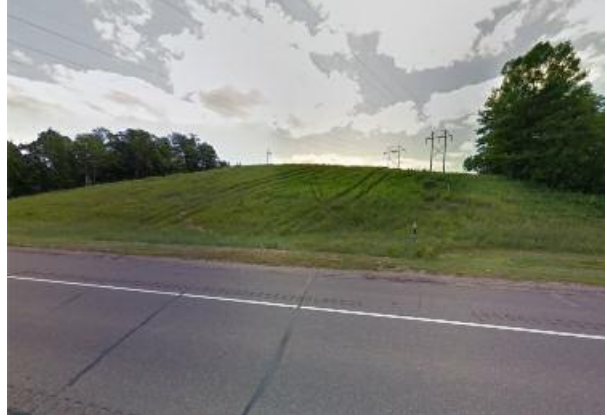
Hwy 210 Looking South at Property
