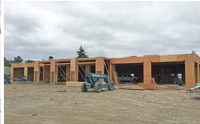
CURRENTLY UNDER CONSTRUCTION
