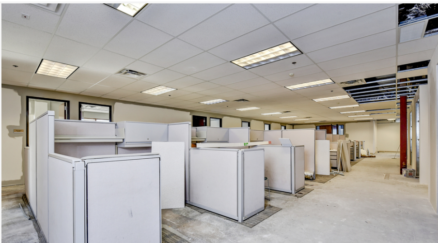
Eagle Home Mortgage: Tenant improvements underway
