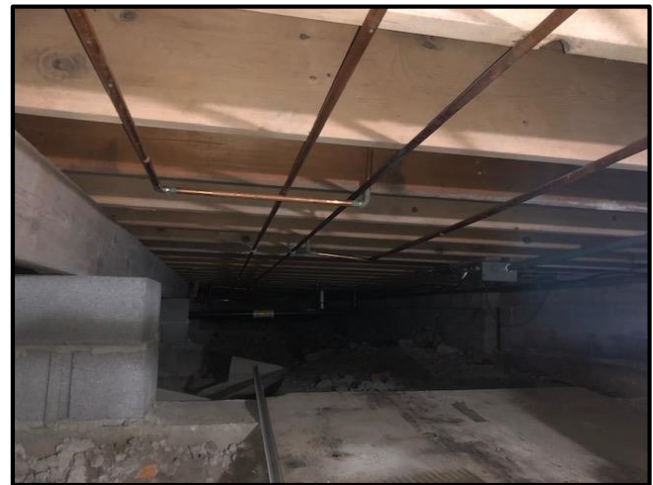
Foundation and basement joist
