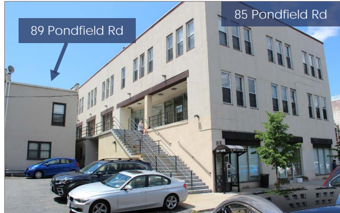
Parking Lot Level + Stairs to Walkway
