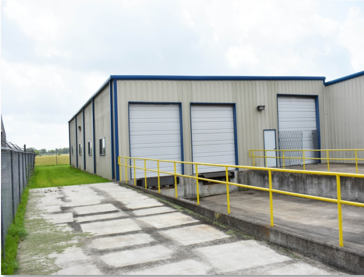
Two Loading Docks
