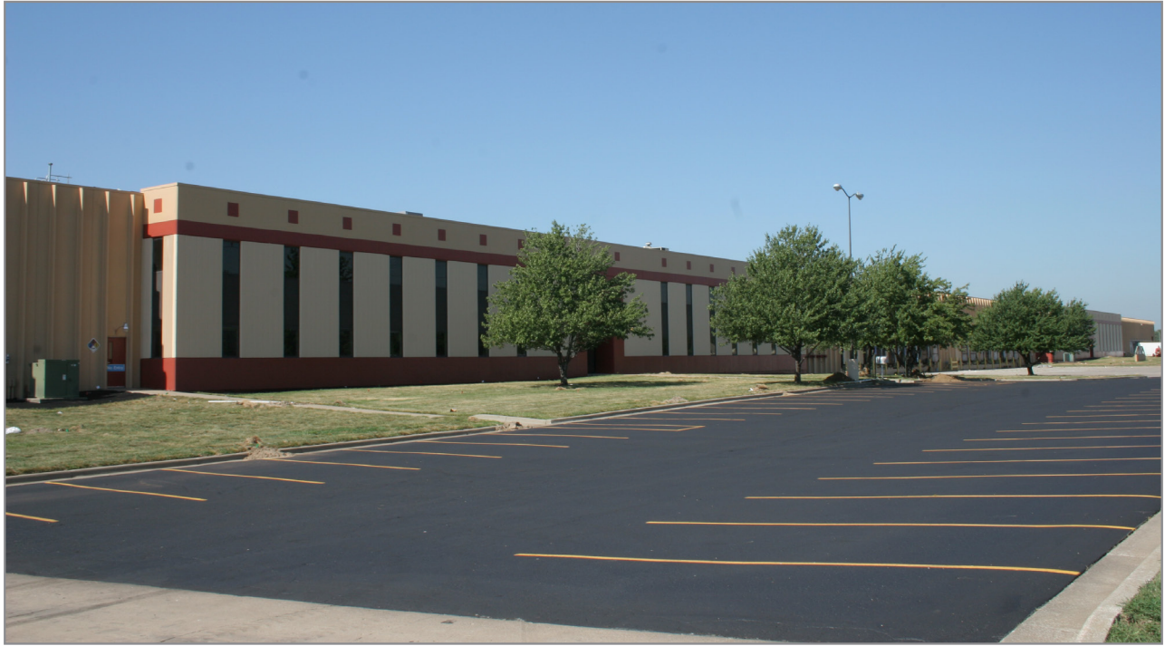
Middle - North Elevation (View NE to SW)
