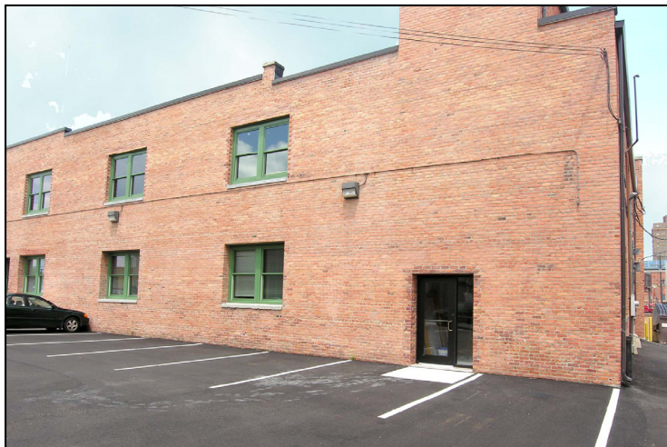
Private suite entrance – East side
