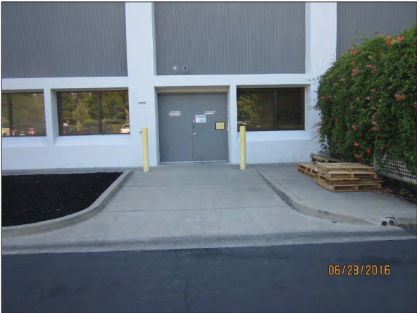
PHOTO OF EXISTING ELEVATION
