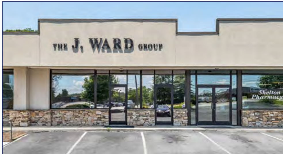
Front, with dual waiting area ingress/egress
