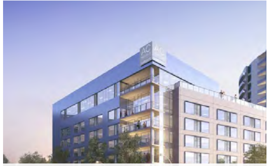
176 room AC Hotels by Marriott under construction
