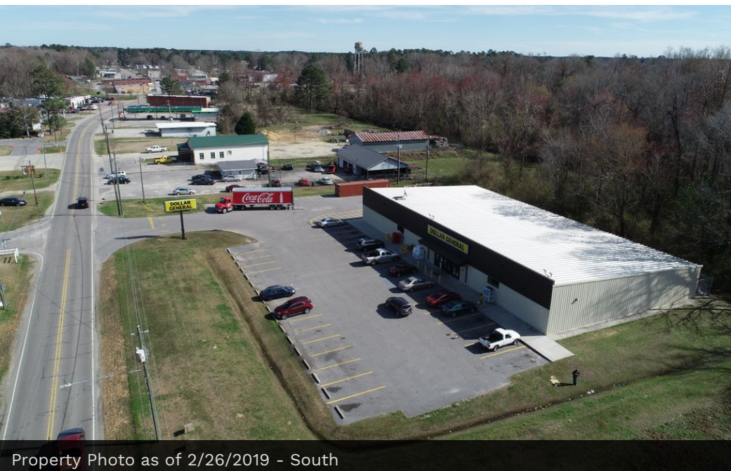
Property Photo as of 2/26/2019 - Southeast
