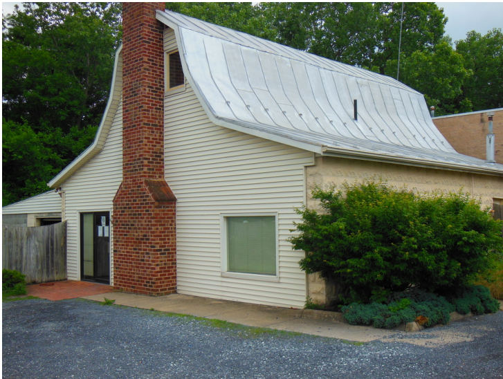
Office building previously leased to ABC Cab Company
