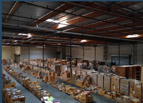
40' x 40' Typical Column Spacing, Skylights with Burglar Bars, Fluorescent Warehouse Lighting
