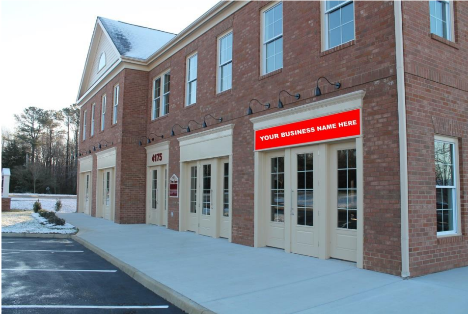
Building Adjacent Parking & Signage Availability
