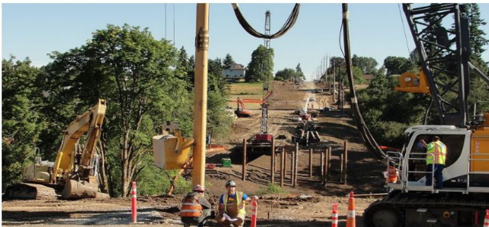
Construction on Northeast 10th
