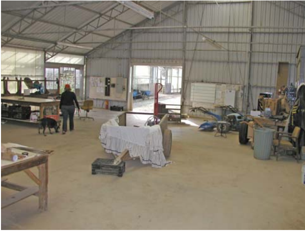
PACKING SHED VIEW #1
