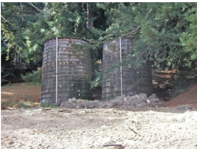
80,000 GAL WATER STORAGE IN 4 REDWOOD WINE TANKS
