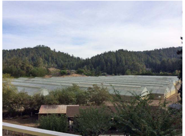
GREENHOUSE VIEW FROM COTTAGE
