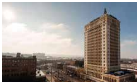
Thomas Jefferson Tower
