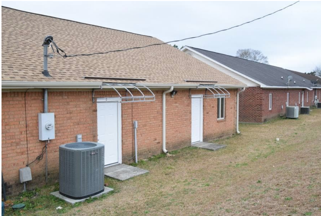
11 3955 1B Rear Exit Doors
