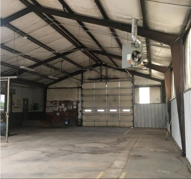
West side of building
