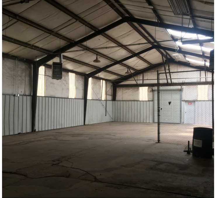
West side of building
