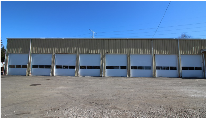
EIGHT 14' H DRIVE-IN DOORS
