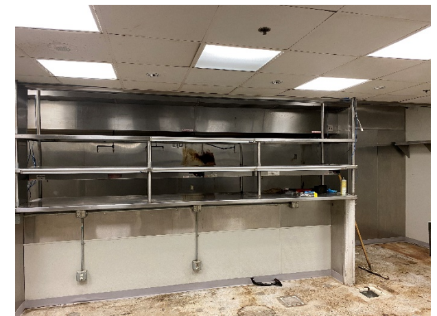
FULL WORKING KITCHEN
