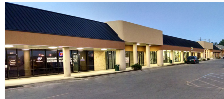
New Strip Renovation
