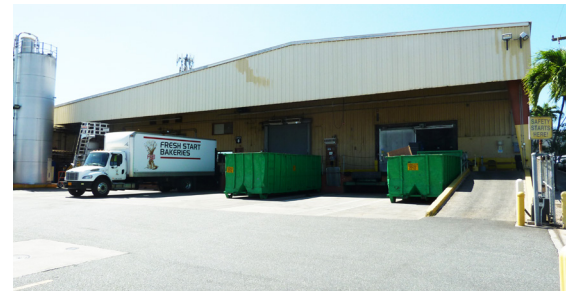
Rear exterior warehouse view
