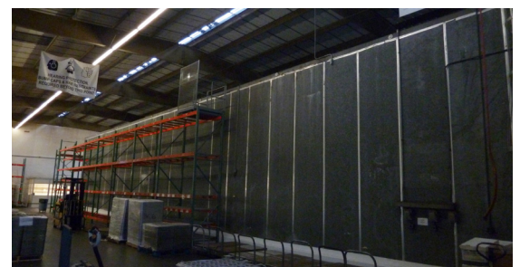
Interior warehouse view
