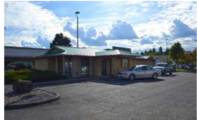
1,564 SF Available Pad Building
