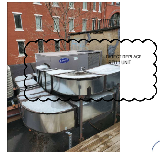
D ROOF CONDENSER LOCATION N.T.S.
