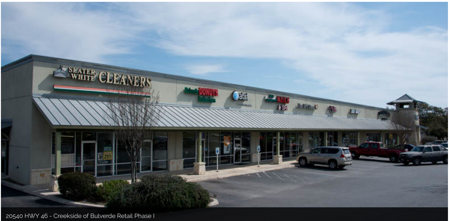
20540 HWY 46 - Creekside of Bulverde Retail Phase I
