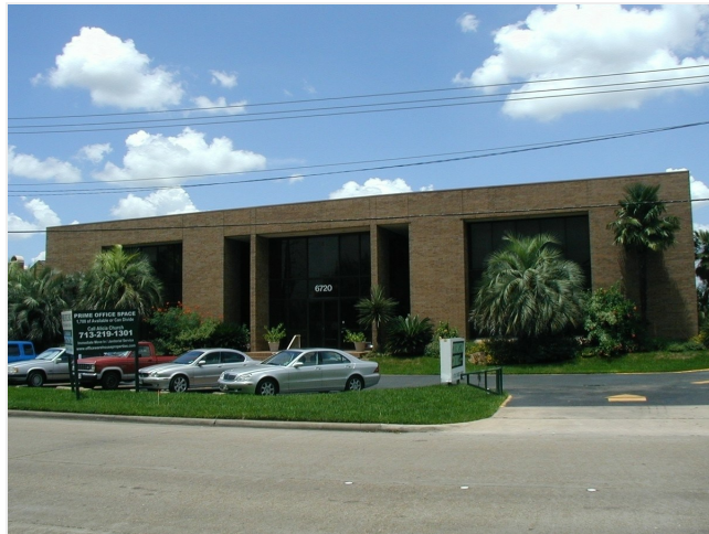
Front of Building
