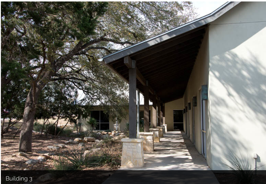
Building 3 184 Creekside Park
