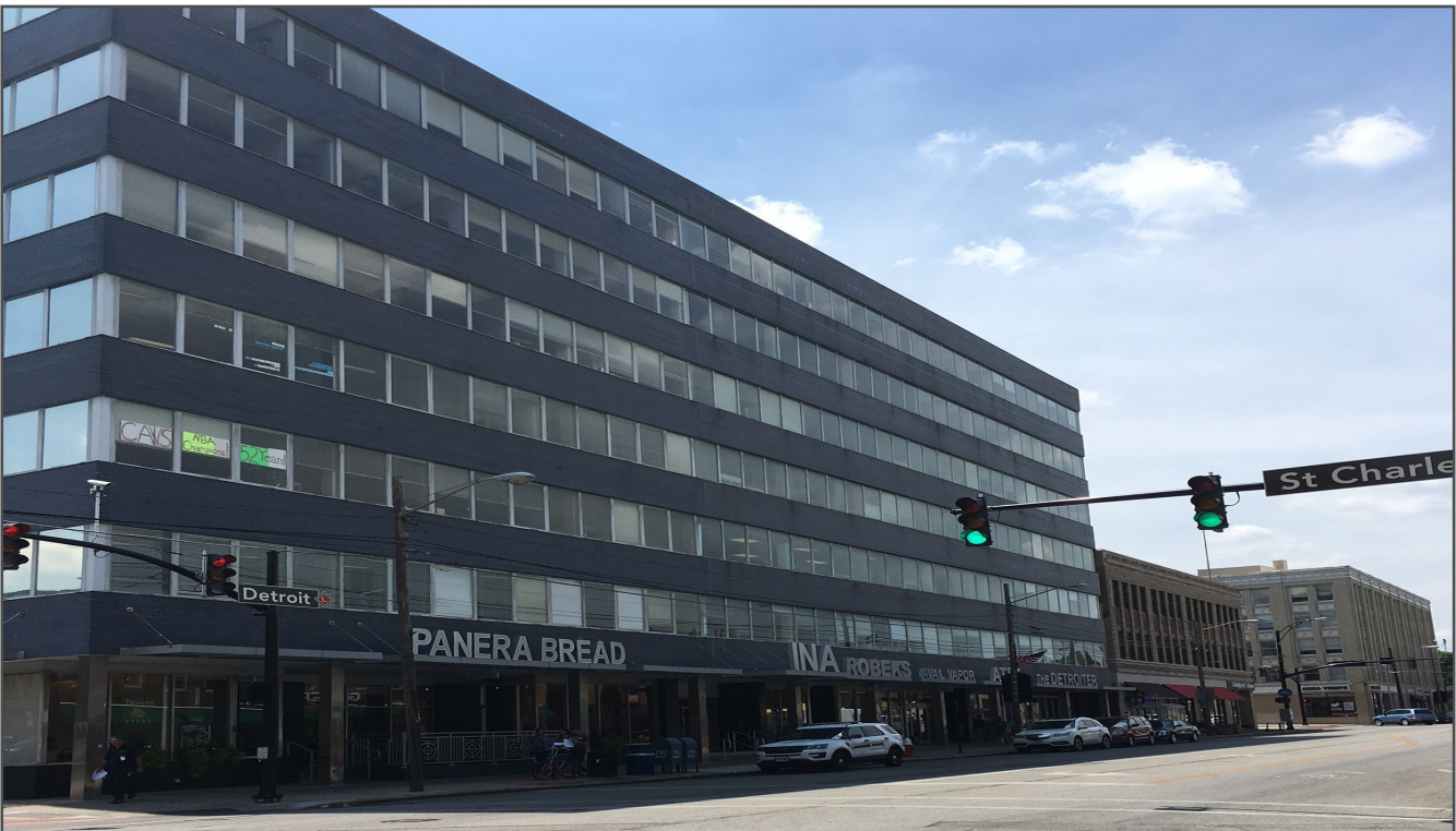
VIEW OF BUILDING
