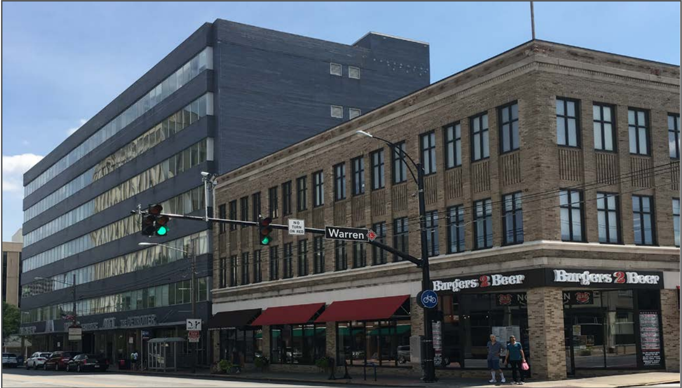
VIEW OF BUILDING
