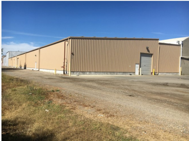
EXTERIOR OF DRY STORAGE
