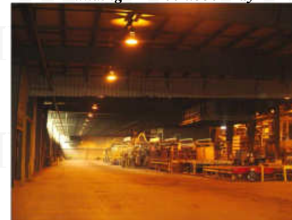
Building #1– 100'x550' Bay
