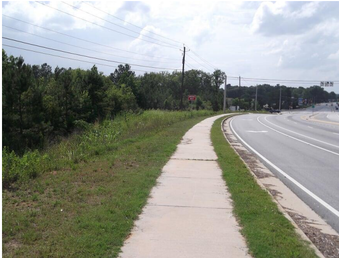
Frontage on Big A Rd. - Sidewalk and Turn Lane
