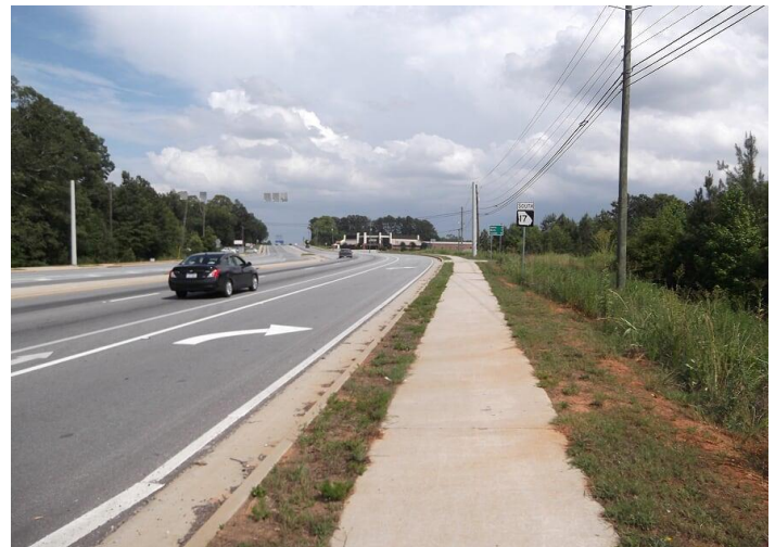
Frontage on Big A Rd. - Sidewalk and Turn Lane
