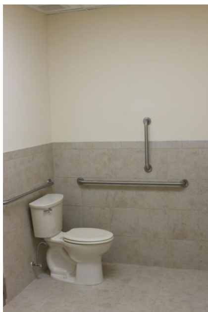
NEW TILE BATHROOM
