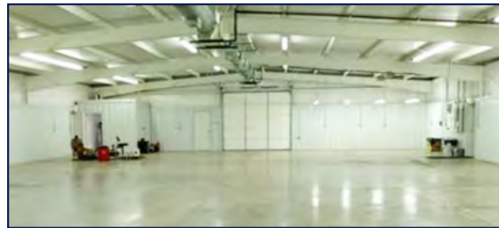
Climate-controlled section, including restroom and shop area
