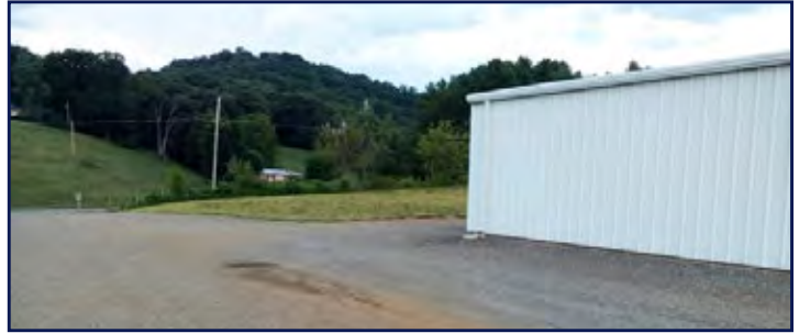
Land is cleared, graded and ready
