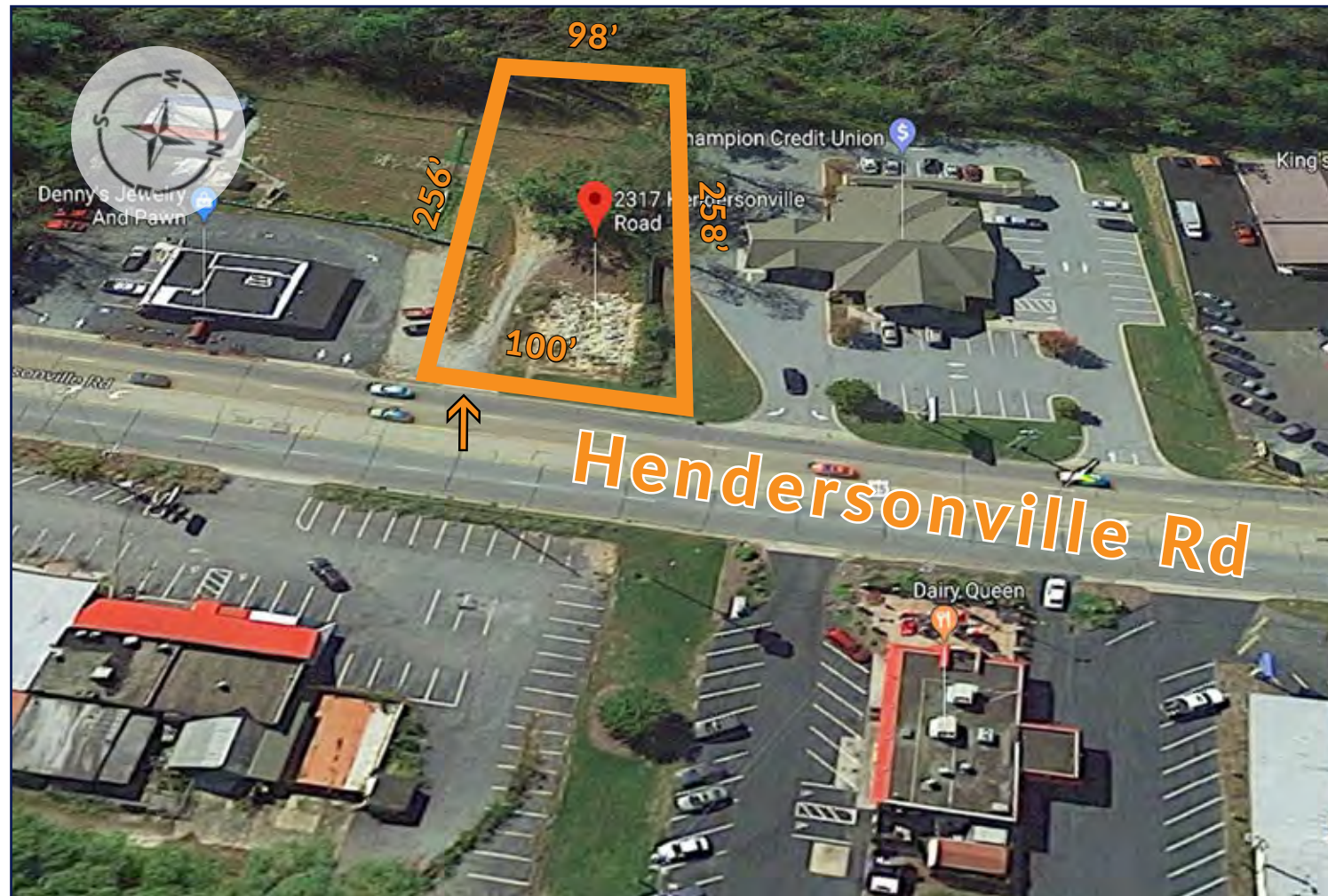
Aerial view looking West
