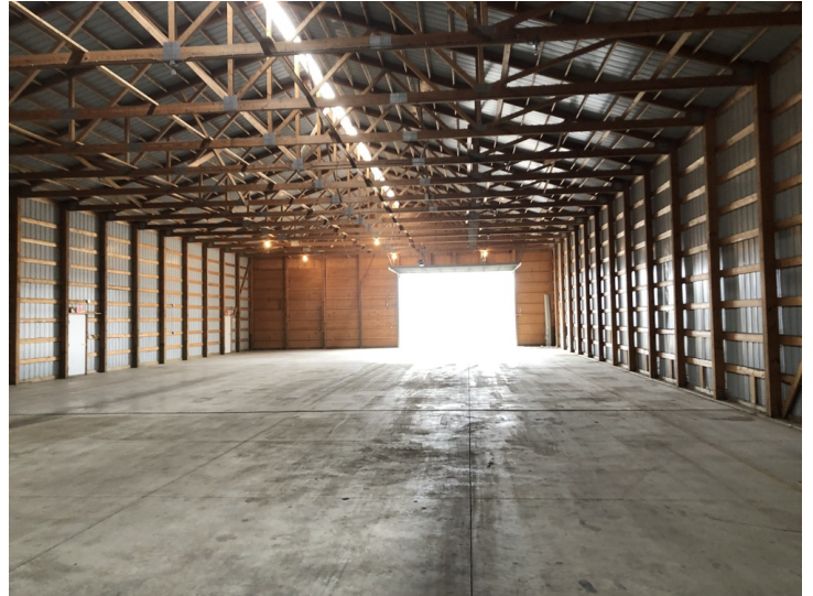
Interior of detached warehouse
