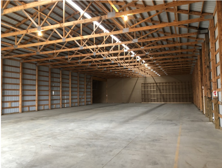
Interior of detached warehouse
