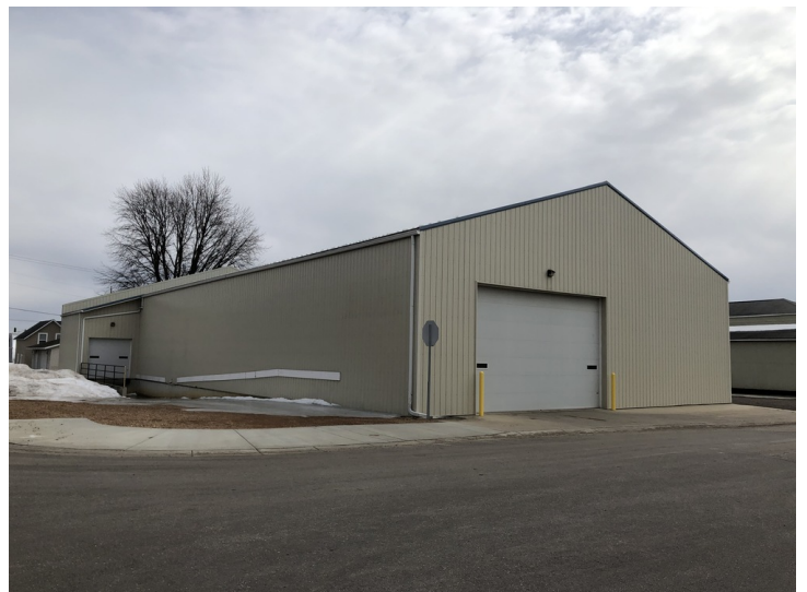
Exterior of detached warehouse
