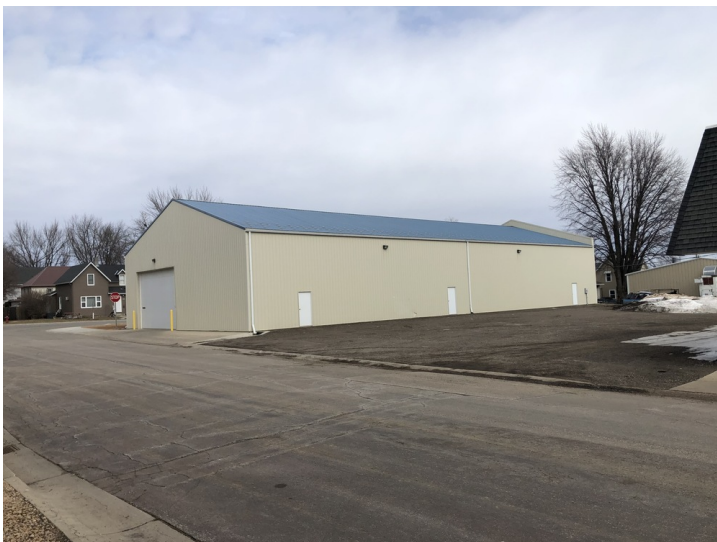
Exterior of detached warehouse
