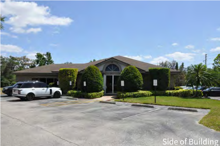
Side of Building
