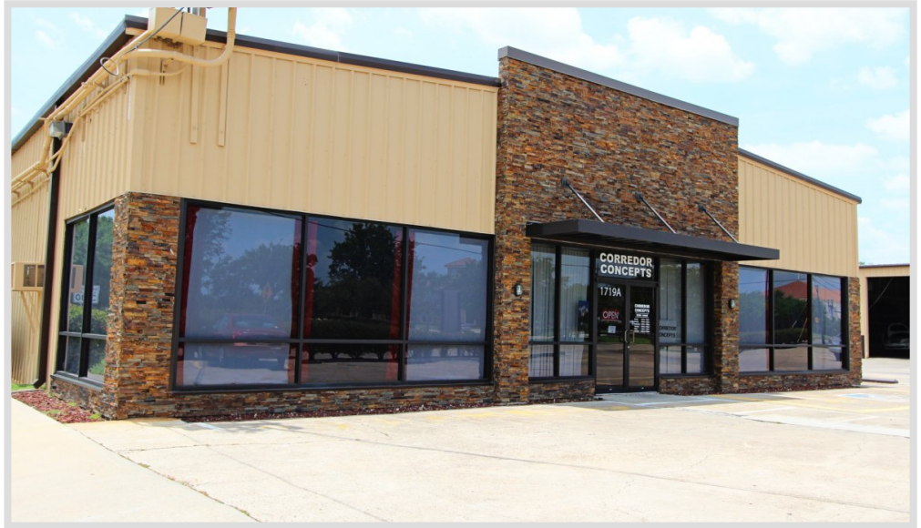
Recently remodeled exterior
