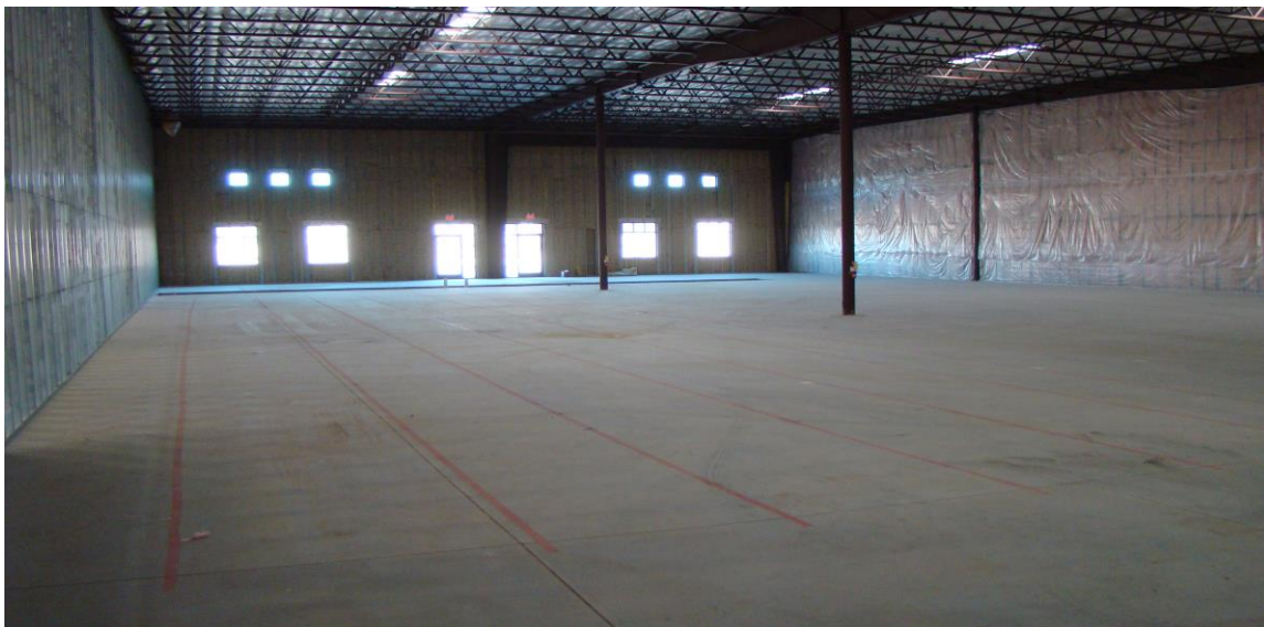
BLDG ANGLE SHOWING BUILDING FRONT ENTRANCE
