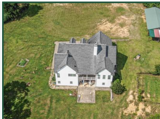
Rear of House
